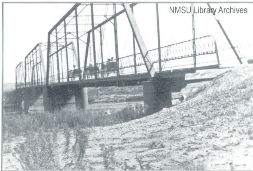
The Rio Hondo Bridge in its original location spanning the Pecos River
