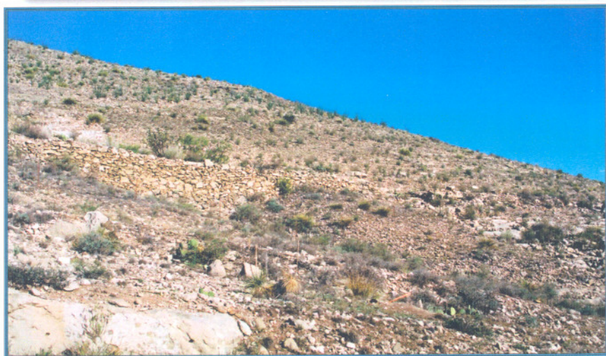
Stone retaining wall between Border Hill and Picacho
