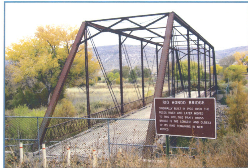
The Rio Hondo Bridge at its current location
